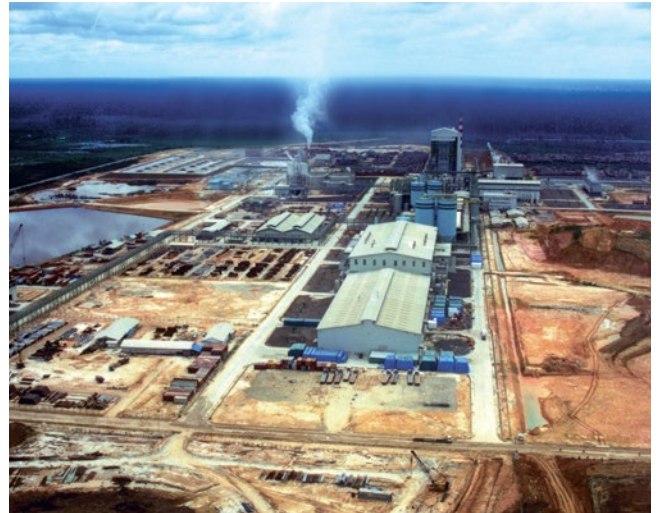
Aerial view of APRIL Pulp Line 1 in 1995. Mill construction adhered to the group's focus on Time, Quality and Cost (TQC), delivering projects faster, better and at more competitive costs.
